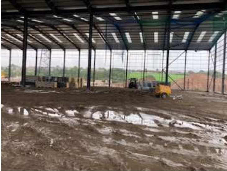
View from rear of building along RoW line showing front elevation
