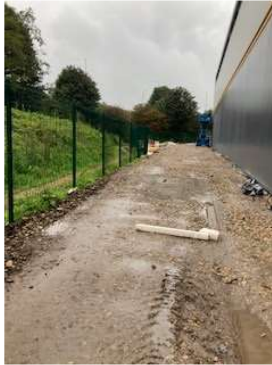
View along side of building back towards steps
